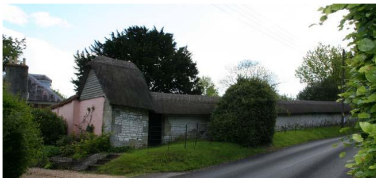
Thatched “block chalk” wall on Stops Hill
