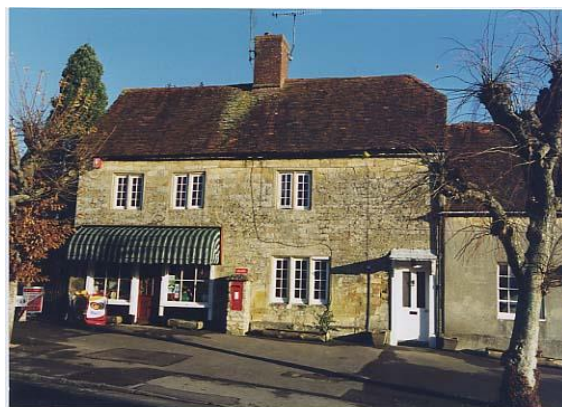
Hindon Post Office and shop
